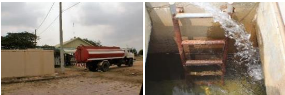
Figure 10: Water Delivery Truck (Left) and Potable Water Holding Tank (Right)
